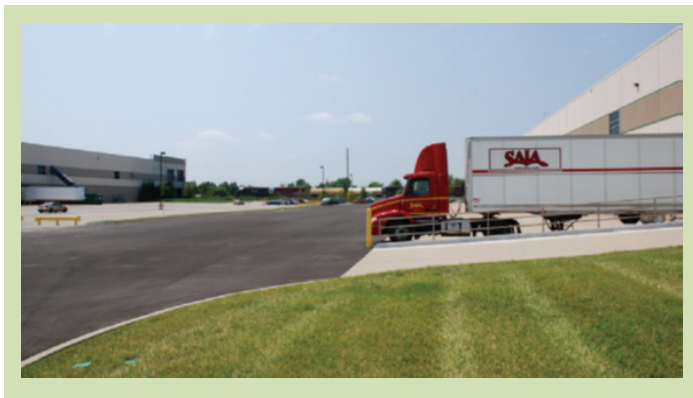
Figure 3.3. Truck Loading Area
