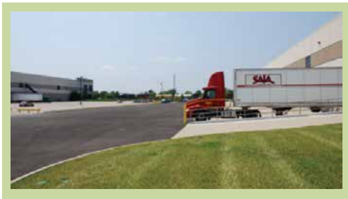
Figure 3.3. Truck Loading Area
