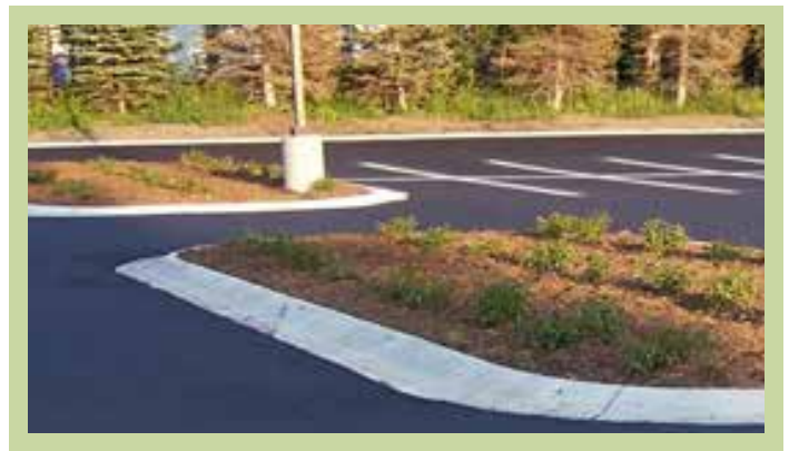
Figure 3.2. Parking lot curbs can be both functional and aesthetic.
